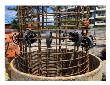
Co-Packers heavy-duty cage wheel spacers guarantee consistent structural integrity in concrete pilings.
